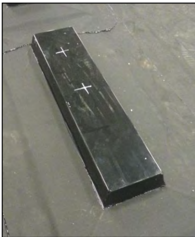
Figure 26: Position hanger bolts on top of hardwood block (covered with aluminium hat)
