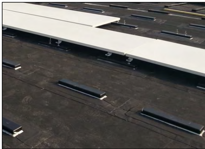
Figure 27: Assembly of GFRC panel with hanger bolts
